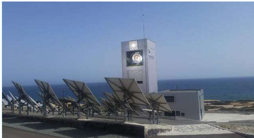
Aspect of Cyl's solar thermal pilot plan for the co-generation of electricity and desalinated water
