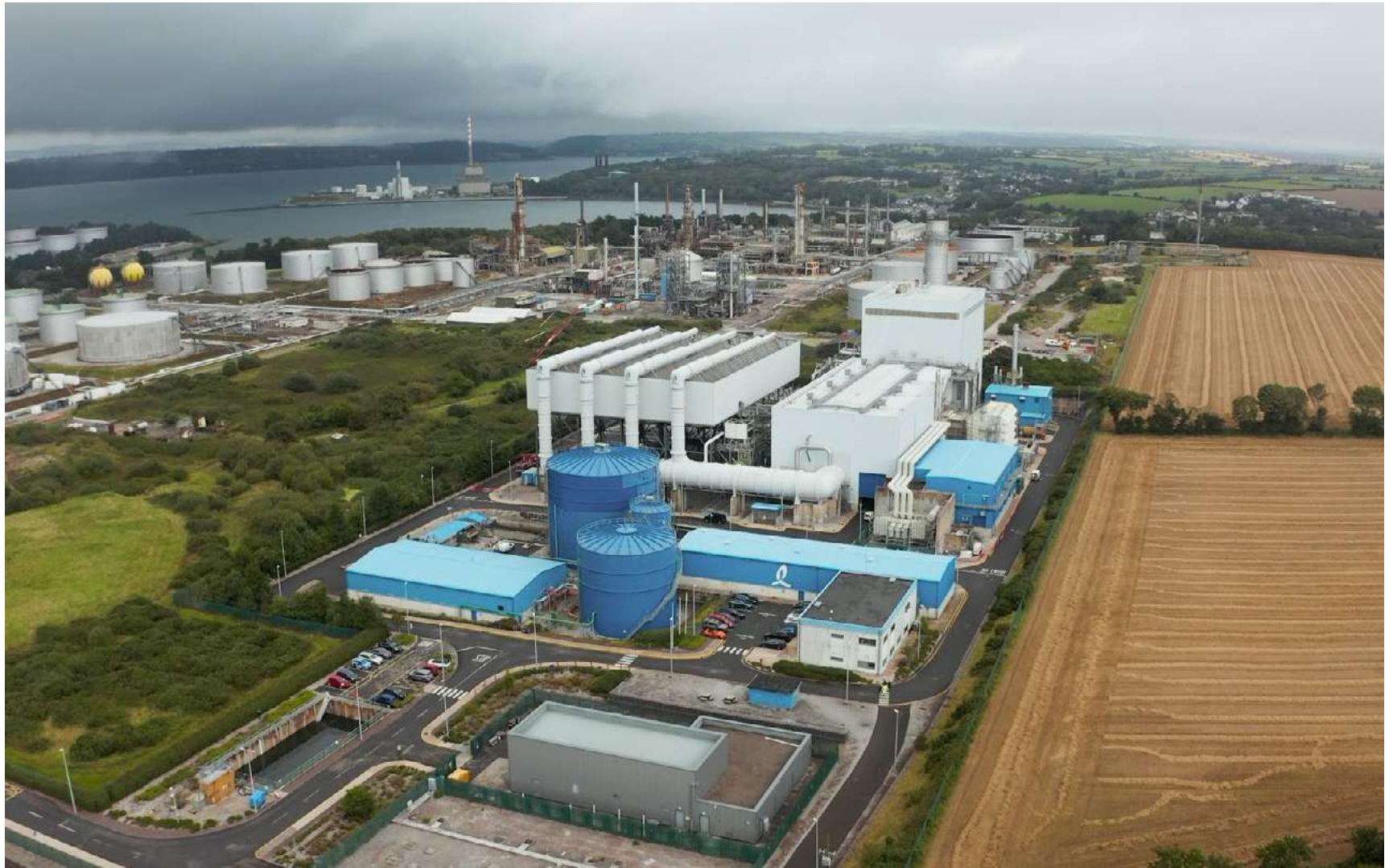
Whitegate Power Generation Plant in Cork
