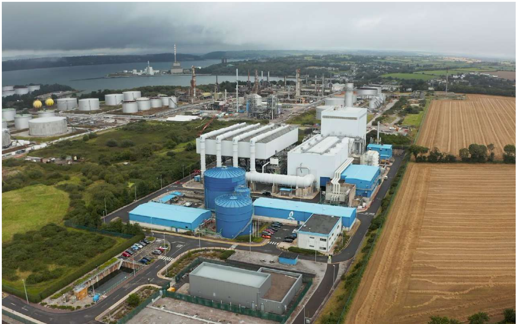
Whitegate Power Generation Plant in Cork
