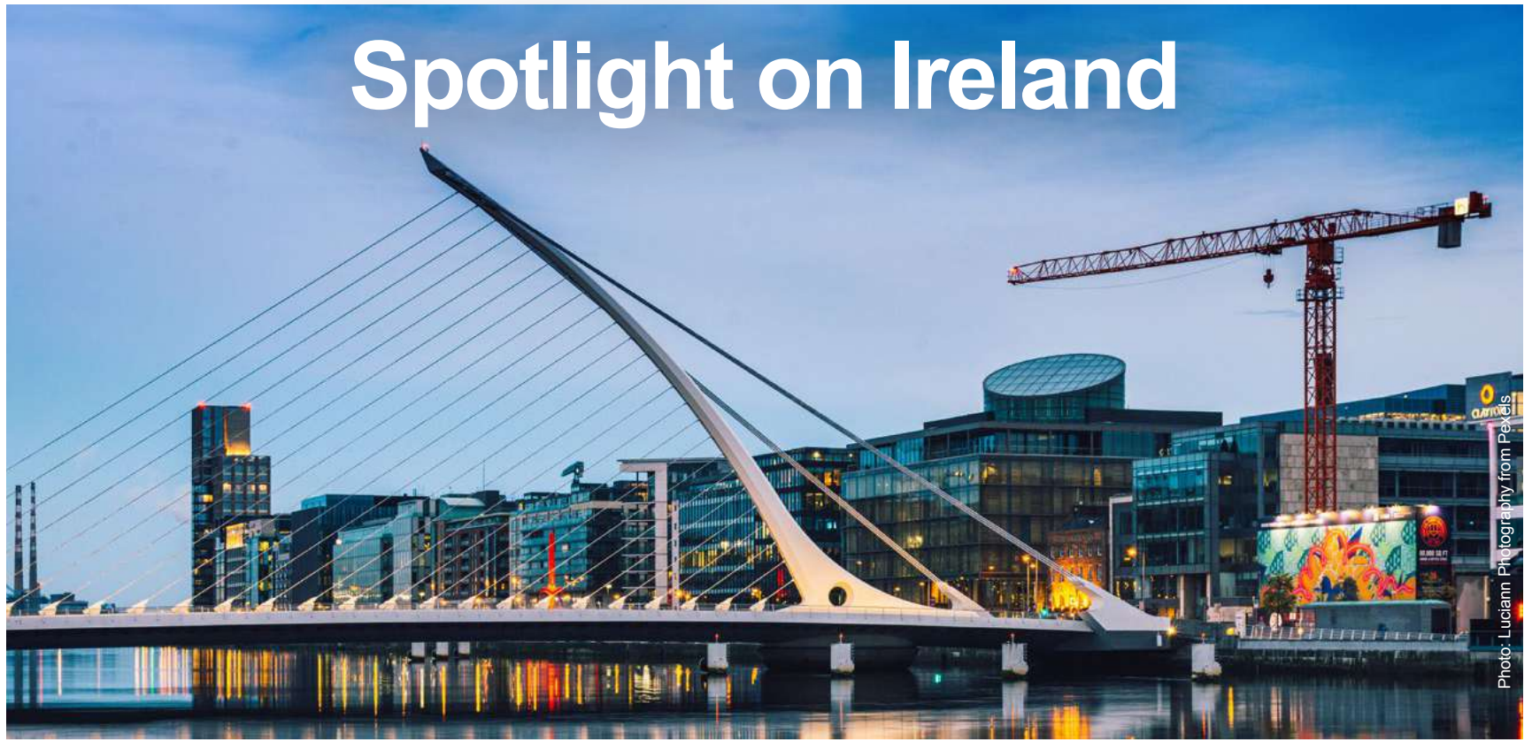
The Samuel Beckett Bridge connects Dublin's Northside and Southside across the graceful waters of the River Liffey within the vibrant Dublin Docklands
